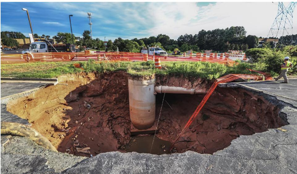
Sinkhole caused by leaking drainage pipe, Gwinnet, County, GA, June 2018
