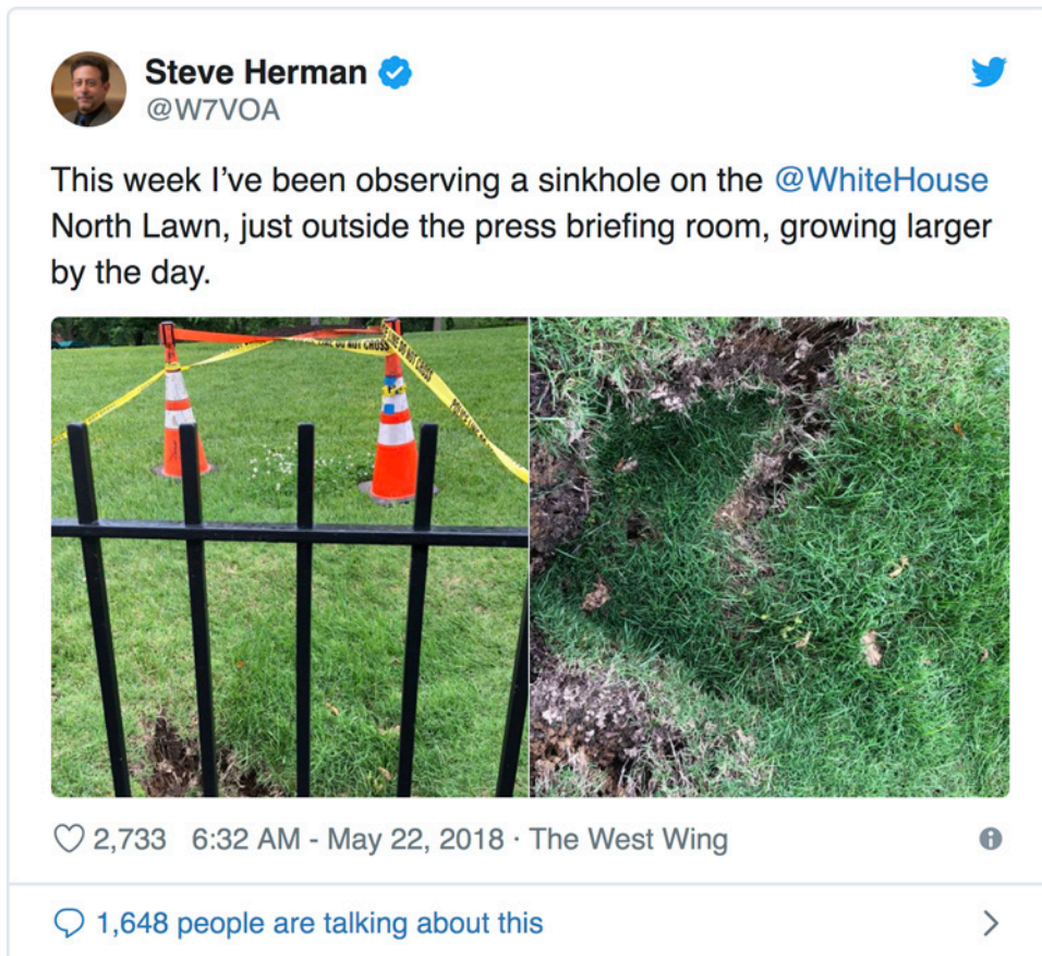
Steve Herman tweets about the White House Sinkhole, May 22, 2018
